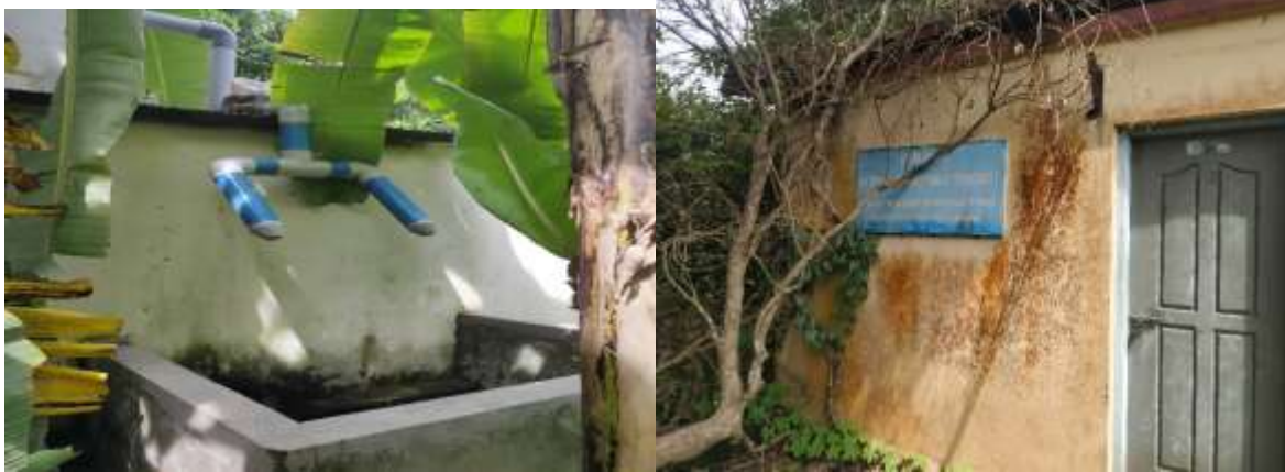
Figure 10RAIN WATER COLLECETION
