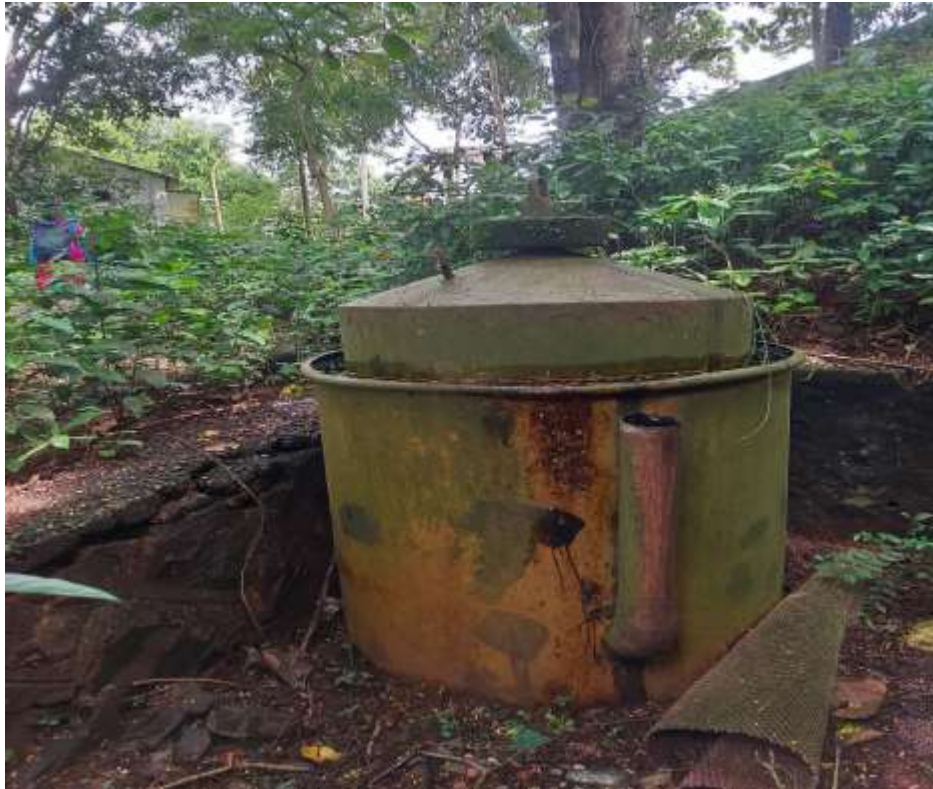
figure 2 FRP BIO GAS PLANT
